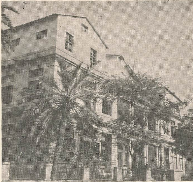
Annexe Building Which houses Principal's Office.
